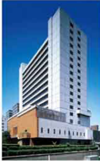
A-2 OFFICE BUILDINGS 銀座MTRビル
